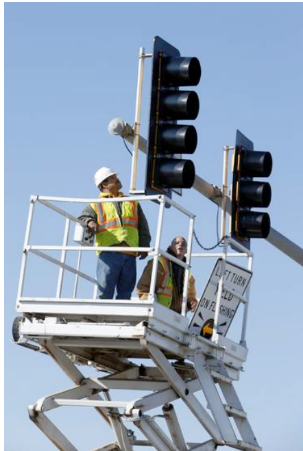
Workers with Traffic Signals, Inc. install a new FYA traffic signal head at Robinson Street and Berry Road in Norman
