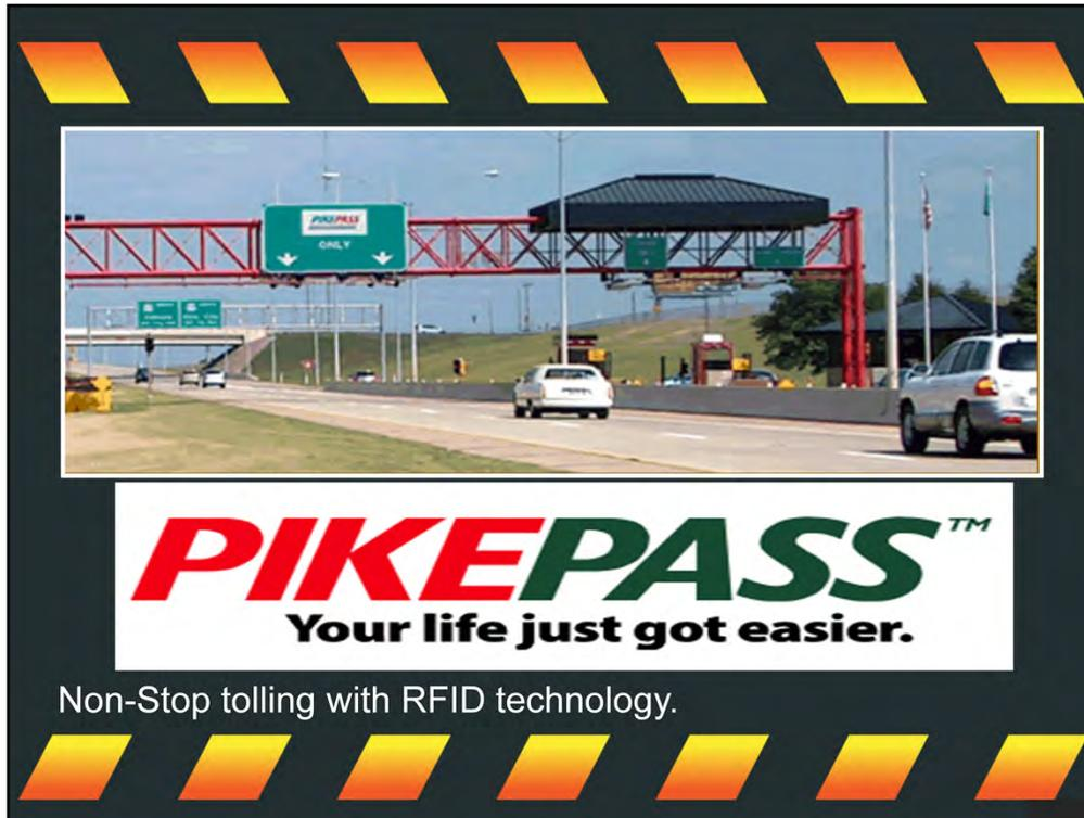
In 1991, the OTA implemented electronic toll collection with the PIKEPASS. This advancement allowed tolling points where a vehicle is not required to stop. The PPS system consists of multiple components that allow for automatic toll processing through the use of RFID technology.
