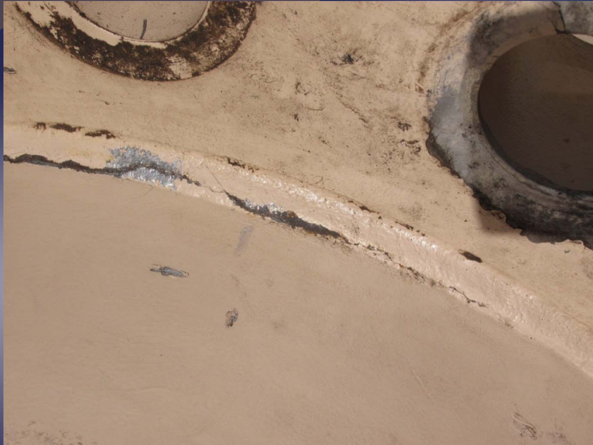
Western Monotube Crack
